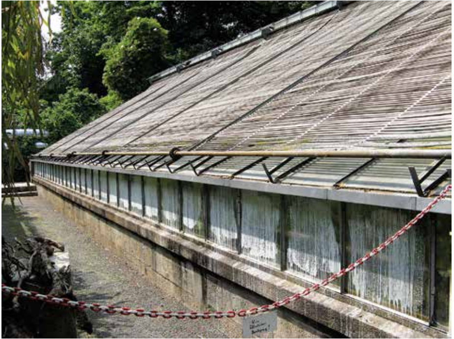
Fig. 5. Greenhouse roof shading. Photo by the author.
