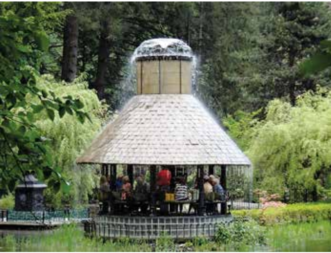
Fig. 7. A 40-foot circular structure in the water room.
