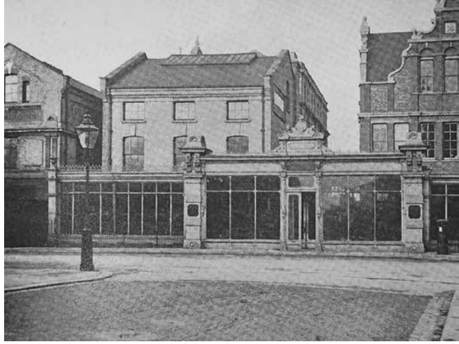
Fig. 8. The main entrance, depot and offices at the Royal Exotic Nursery at Chelsea.
